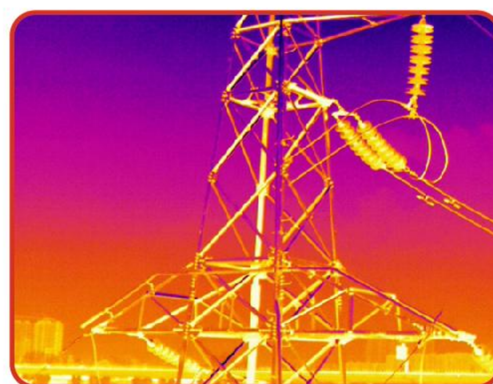
Power operation and inspection
